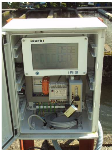
Outdoor (IP66) cabinet tailored telecontrol outstation in a plug & play industrial execution.
