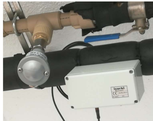
⇐ ↑ ISURLOG 2 on-field unit for HVAC network temperatures monitoring at a health facility.
