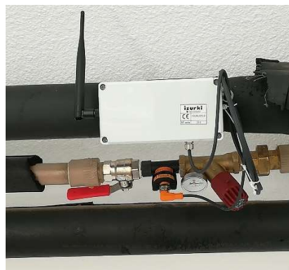
ISURLOG-LR deployed unit remotely monitoring flow and temperature on a hot water distribution network with LoRa comms.
